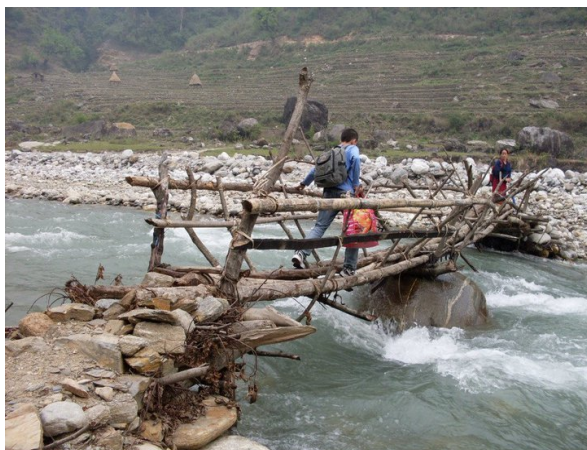
Figure 6. Temporary bridge in the Madi river after the suspension bridge has been washed away.
